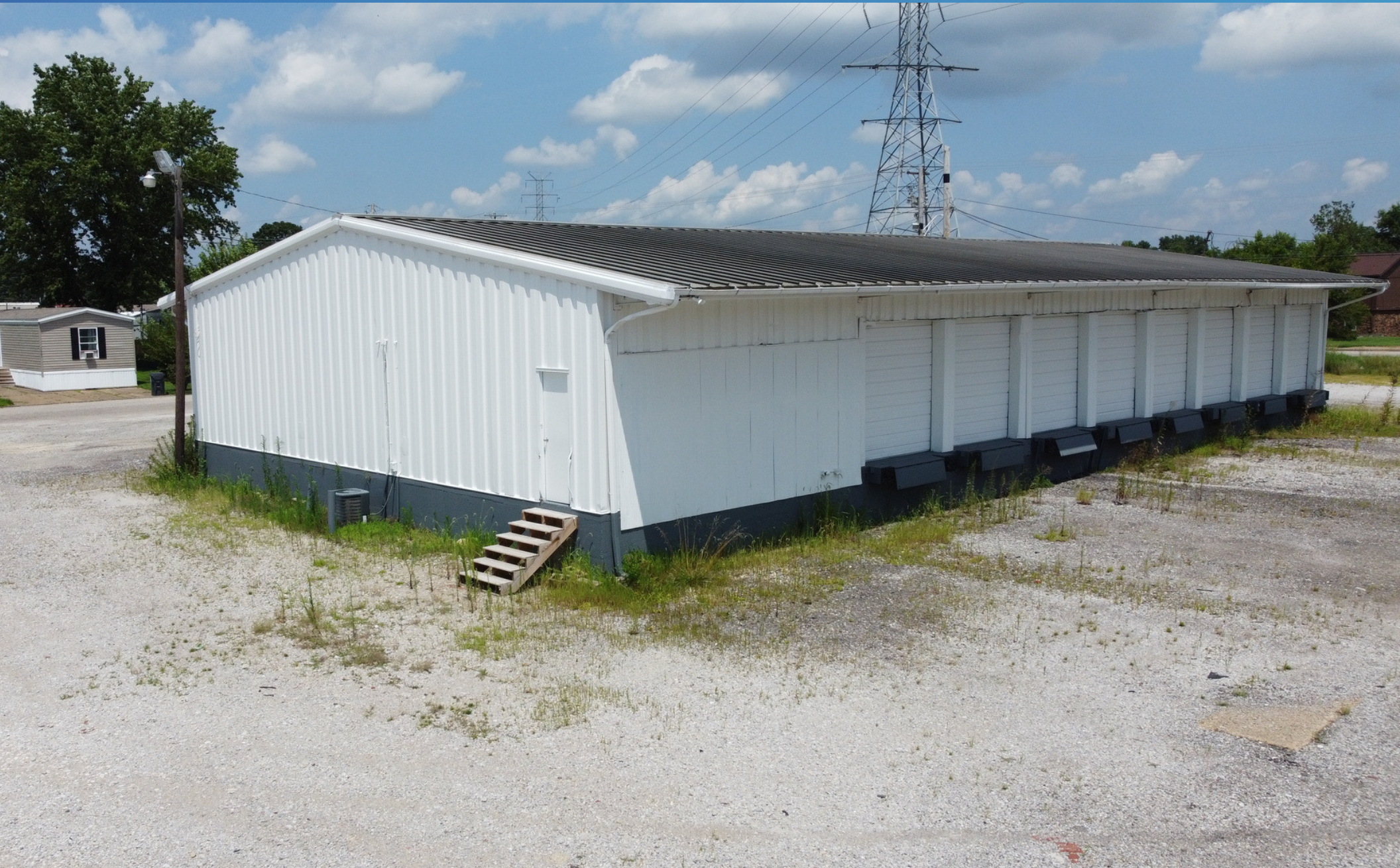
2780 Kratzville Building - 16 Door Cross Dock Terminal - Southside
