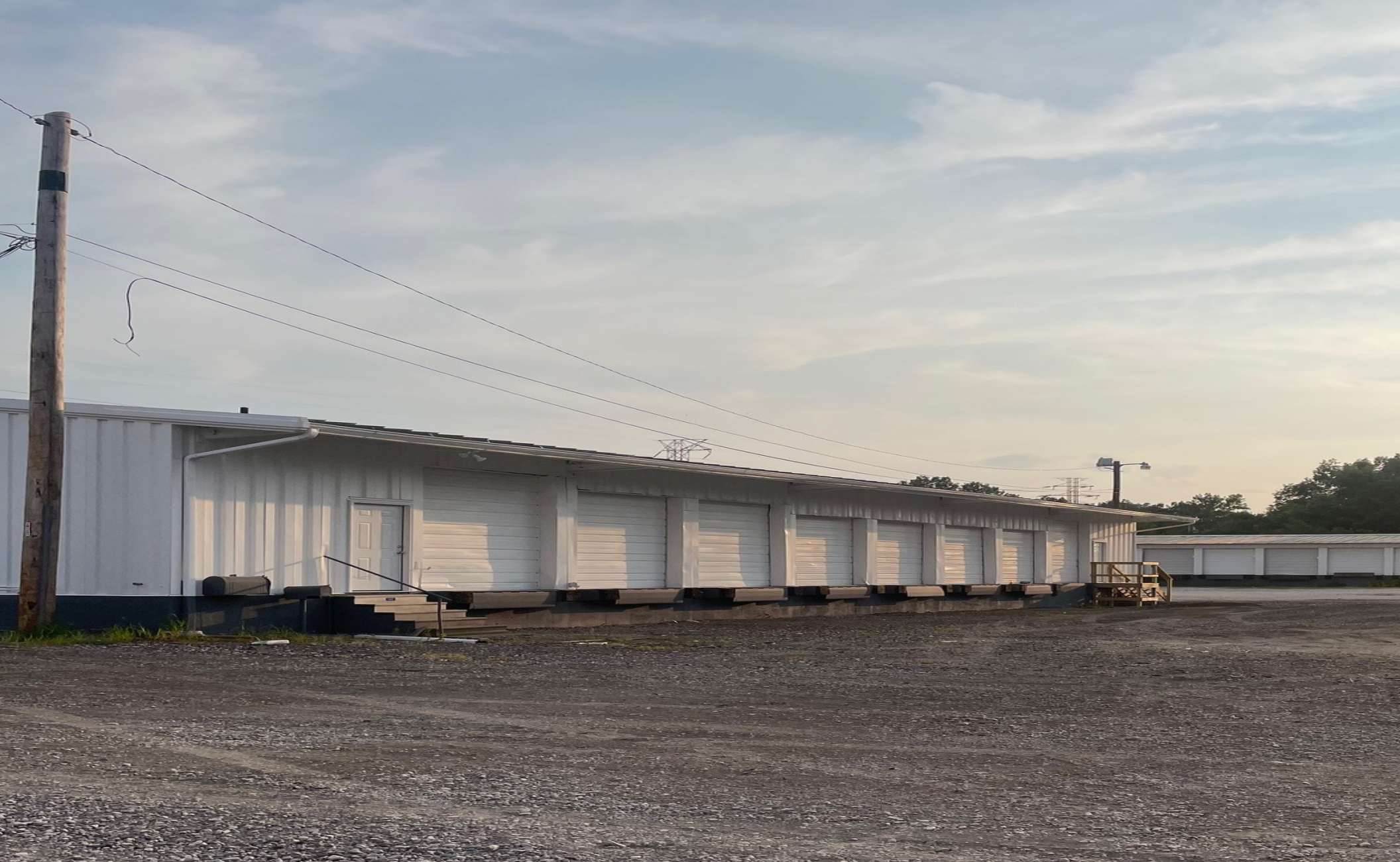
2780 Kratzville Building - 16 Door Cross Dock Terminal - Northside
