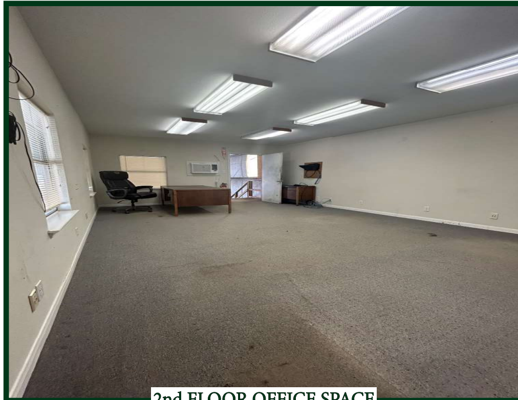
2nd FLOOR OFFICE SPACE
