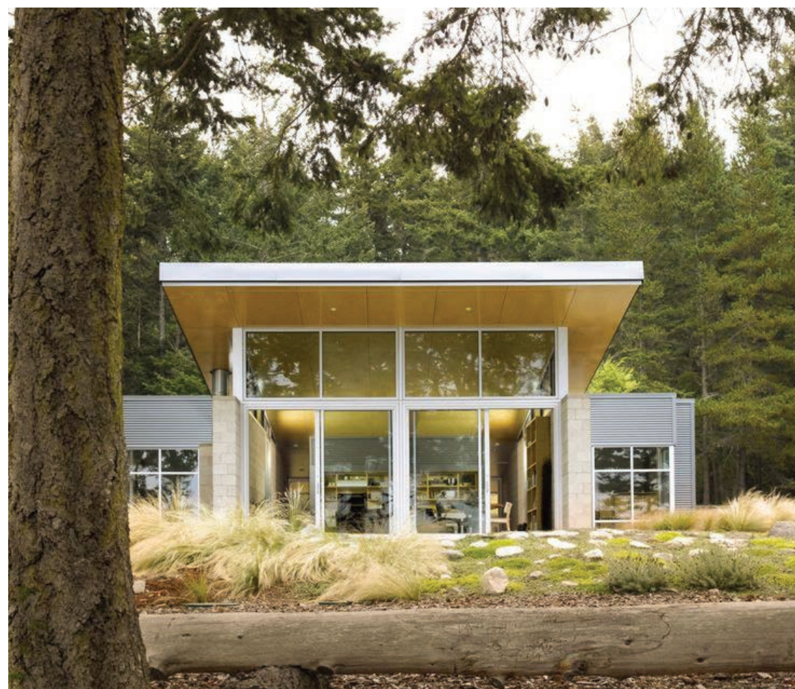
Modern Single Sloped Roof Structure
