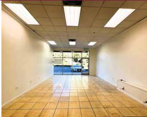
Interior - Upgraded Tile Flooring Throughout
