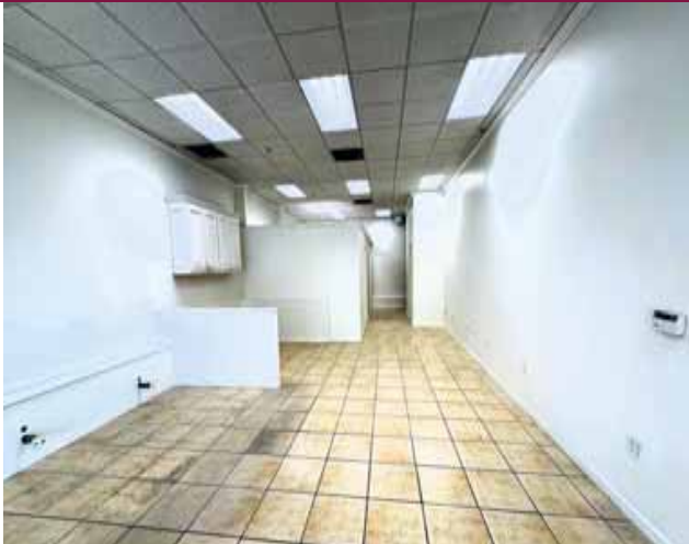
Interior - Plumbing Stub Outs for 6 Shampoo Bowls
