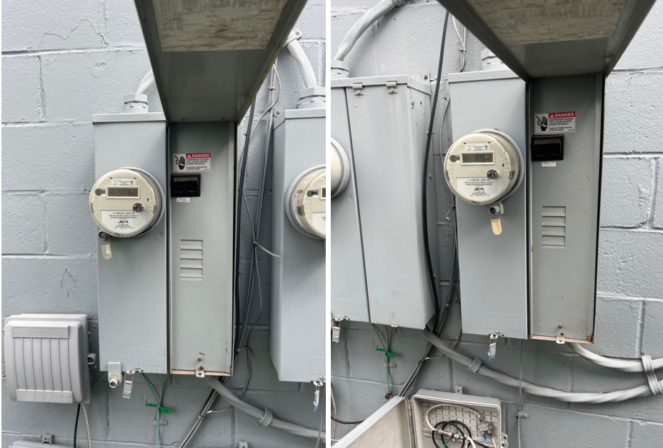
General Info: Service Amperage 150amps 120/240VAC
