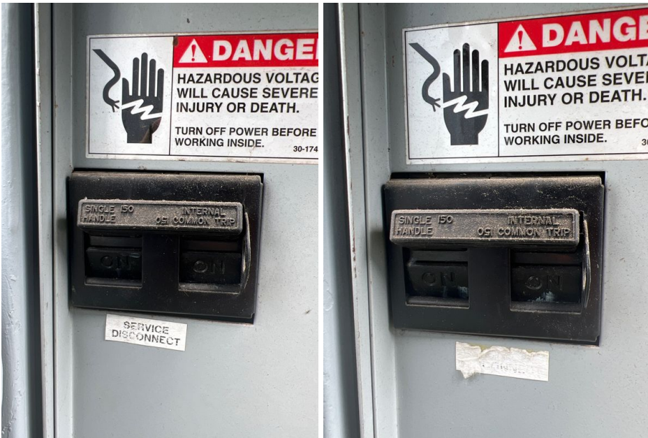
General Info: Service Amperage 150amps 120/240VAC
