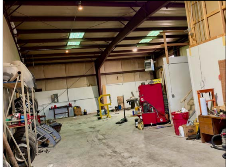
Service bay • 16' walls, clear-span steel frame
