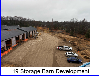
19 Storage Barn Development
