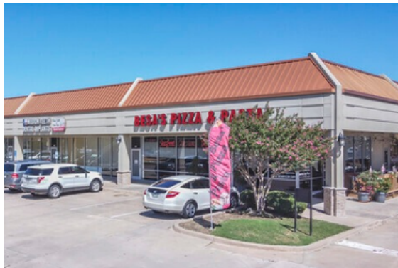
14856 PRESTON ROAD BUILDING 1
