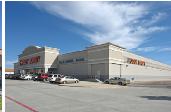
14858 PRESTON ROAD BUILDING 3 | HOBBY LOBBY
