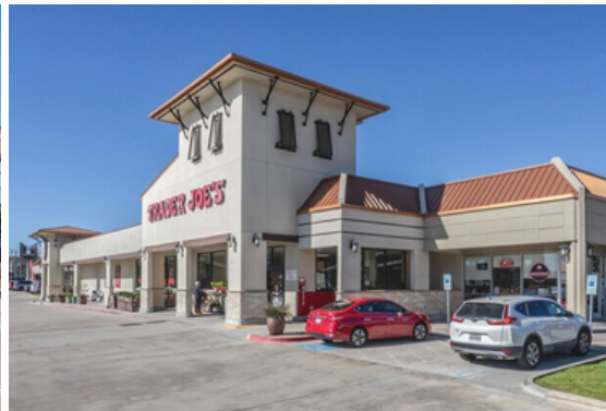
14856 PRESTON ROAD BUILDING 2 | TRADER JOES
