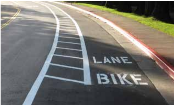
On-street bicycle facilities include bike lanes and other facilities that are located within the street right-of-way.
