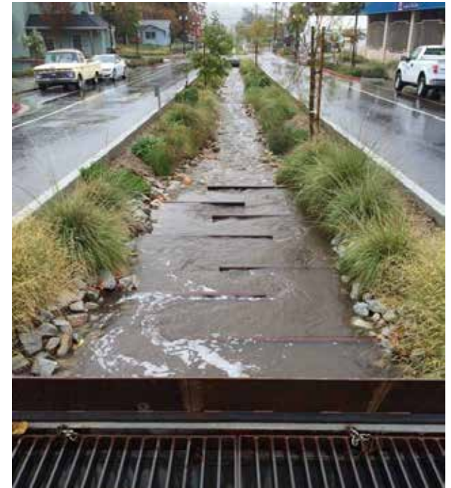
A central channel concept similar to the one pictured above could be used in conjunction with the inverted crown of West Elkhorn to assist with the capture and conveyance of storm flows and flood water.
