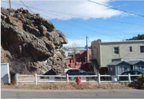
Existing outcropping blocking the proposed Cleave Street extension (from reverse angle as shown above in Figures 5.14 and 5.15).
