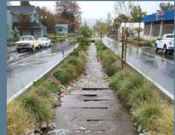
A central open channel collects and conveys storm flows away from buildings.
