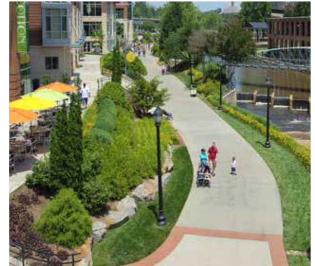
Terraces can serve outdoor recreation during normal flows, but convey water during flood events.
