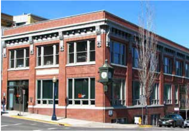
An eclectic mix of traditional and contemporary buildings should mix with existing ones along Elkhorn Avenue.
