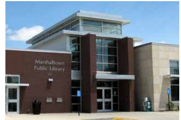
Redevelopment of the Town Hall site should include civic uses.
