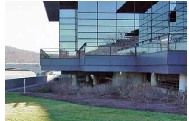
A building could include parking on lower levels that is designed to absorb and permit water flow during flood events.
