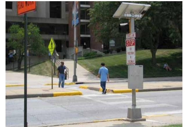
Pedestrian refuge islands can be integrated into midblock crossings. (Source: USDOT Federal Highway Administration)
