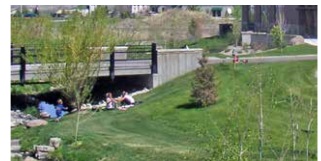
Terraced walls and flood detention areas can also provide passive recreation amenity spaces during times of low water flow.
