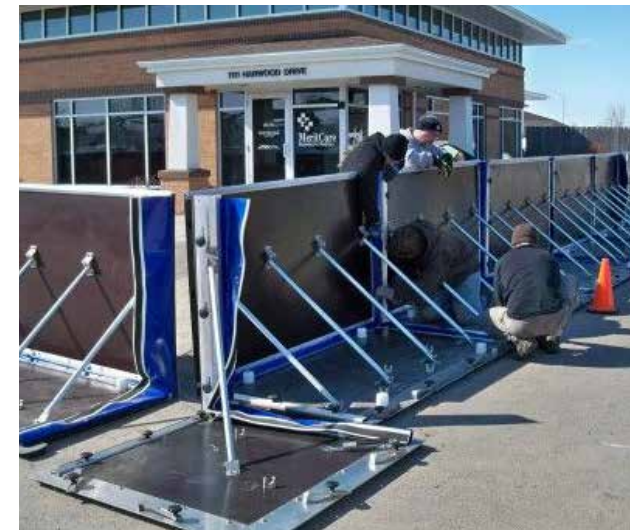
Temporary barrier systems can be erected at times of rising water to protect storefronts and building entries.
