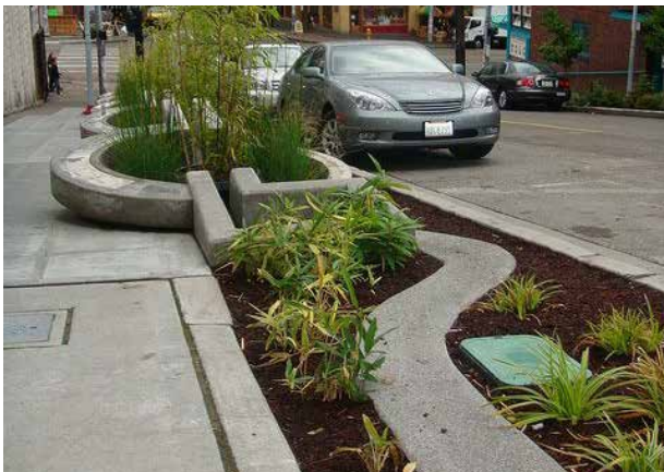
Rain gardens collect and treat runoff from storm and snow events.
