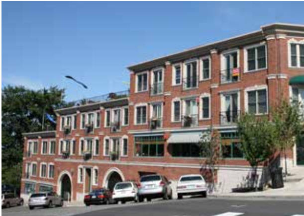
Vary the mass of a building to step with changes in landform.
