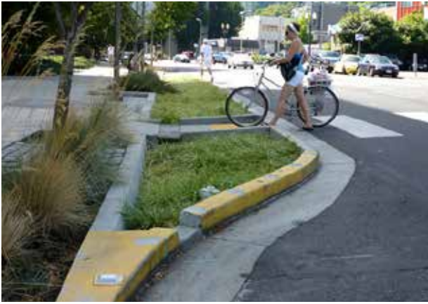
Pedestrian circulation should be enhanced with crossing improvements. Curb extensions or 'bulb-outs' increase pedestrian visibility and decrease pedestrian crossing time. The 'bulb-out' pictured above also includes a curb-cut to collect water from storm flows and snow melt.
