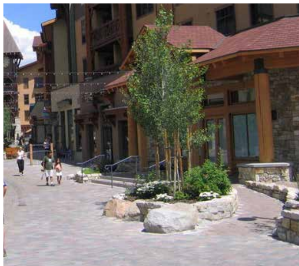
Orient a building to face a street, plaza or the Riverwalk. Residential entries and balconies can also help activate the public realm.
