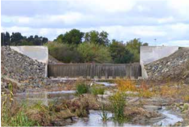
Flood control dams are used to store flood waters and attenuate peak flows.
