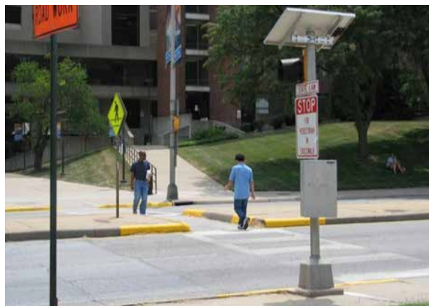
Pedestrian refuge islands can be integrated into midblock crossings. (Source: USDOT Federal Highway Administration)
