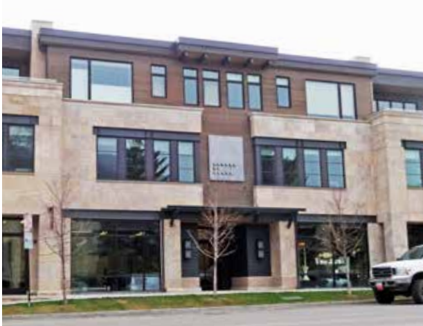
Mass variation techniques include stepbacks, increased setbacks and wall offsets.
