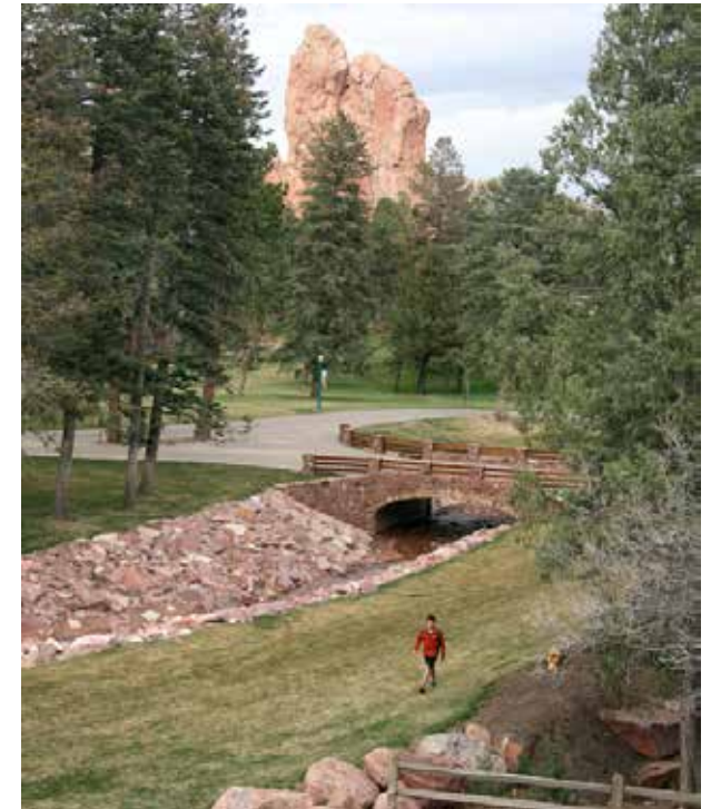
This image shows an example of a widened waterway channel that would be appropriate in the outer areas of Downtown.
