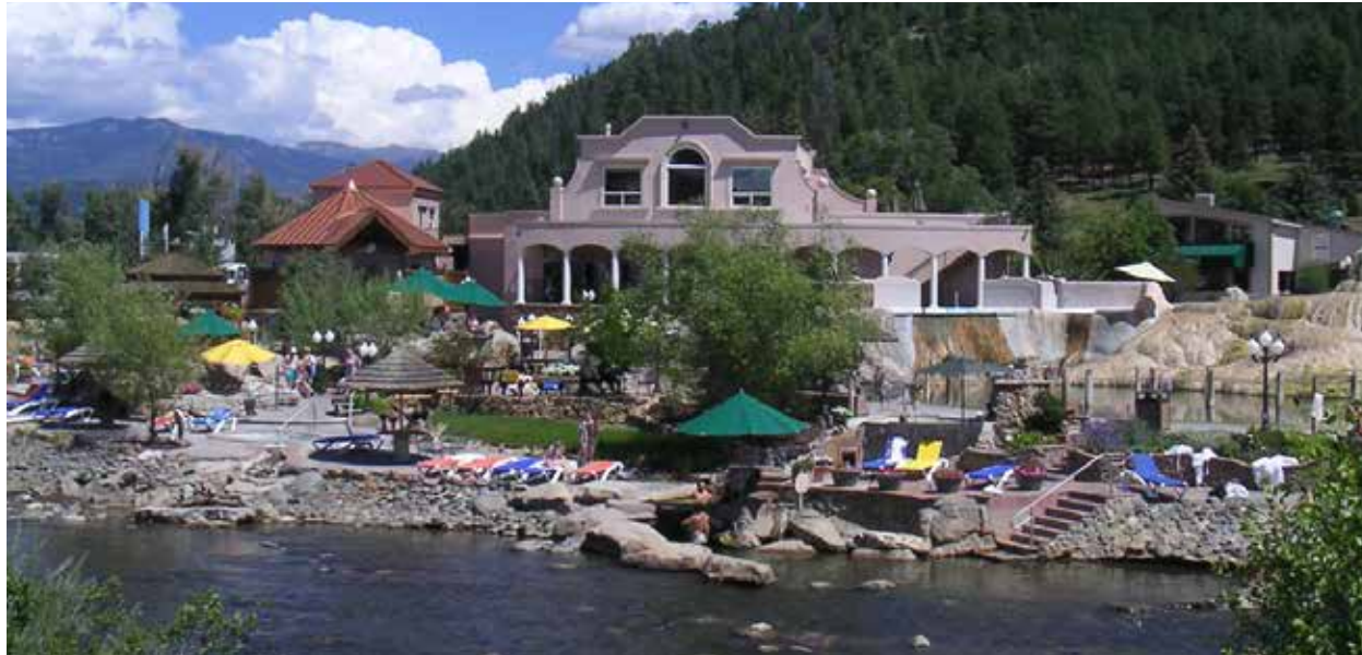
Redevelopment of the Elkhorn Lodge site should consider opportunities to combine river side park space with flood mitigation improvements, such as channel benching as seen in this image.
