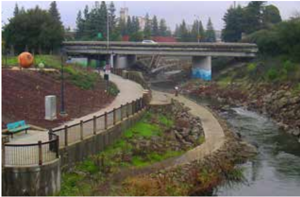
Multi-use trails can aid in flood conveyance.
