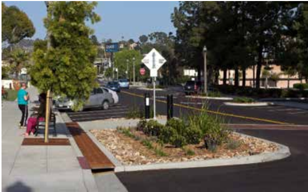
Landscaped parking islands capture parking lot runoff and provide water quality treatment and infiltration.
