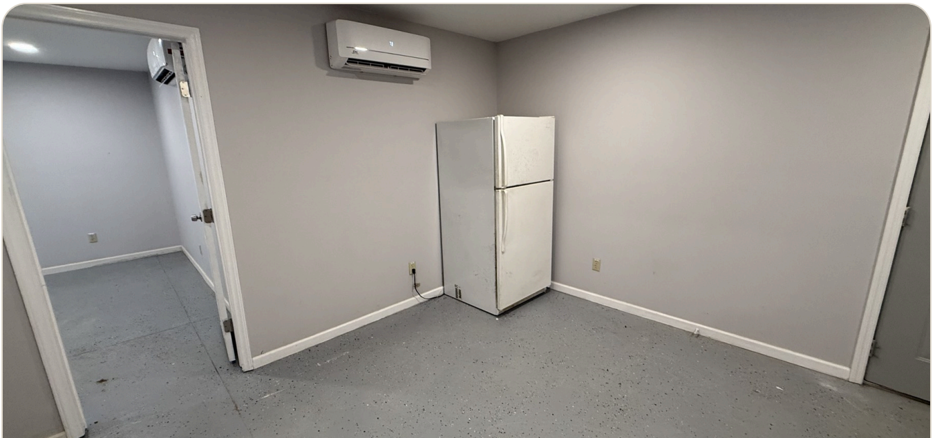
Finished HVAC office/support space
