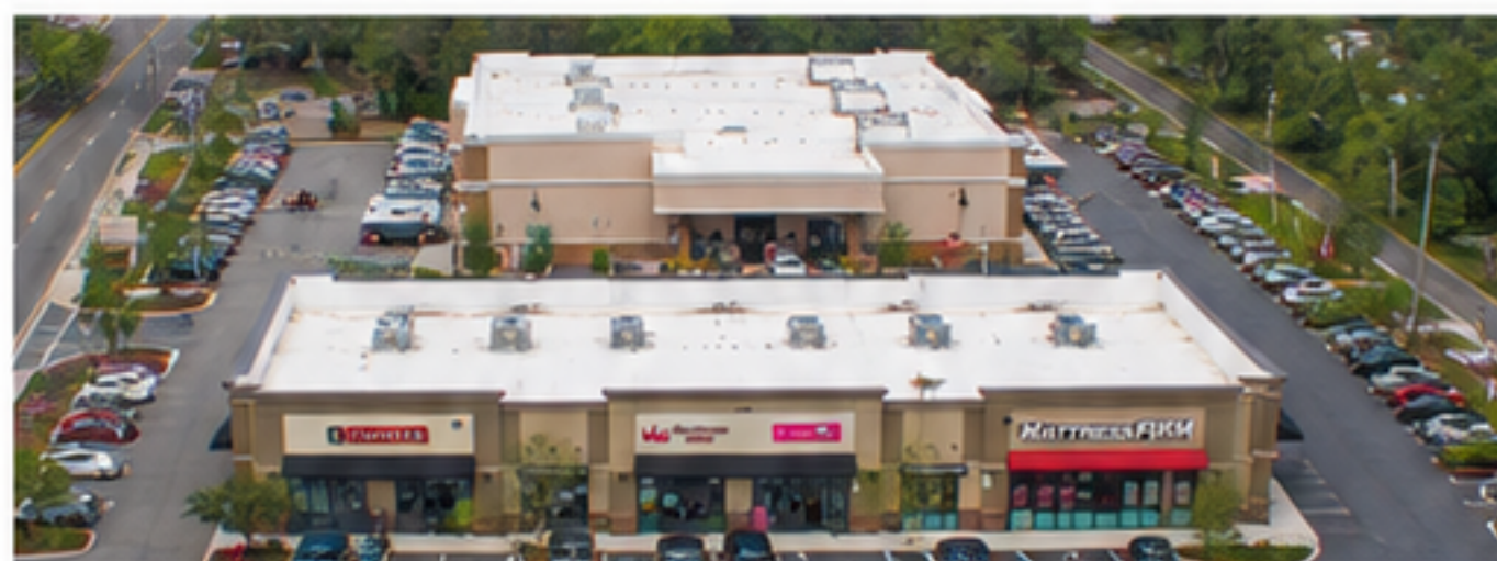
CENTER AERIAL — NW 13 TH ST FRONTAGE
