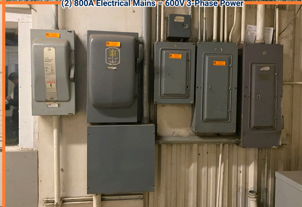
(2) 800A Electrical Mains - 600V 3-Phase Power
