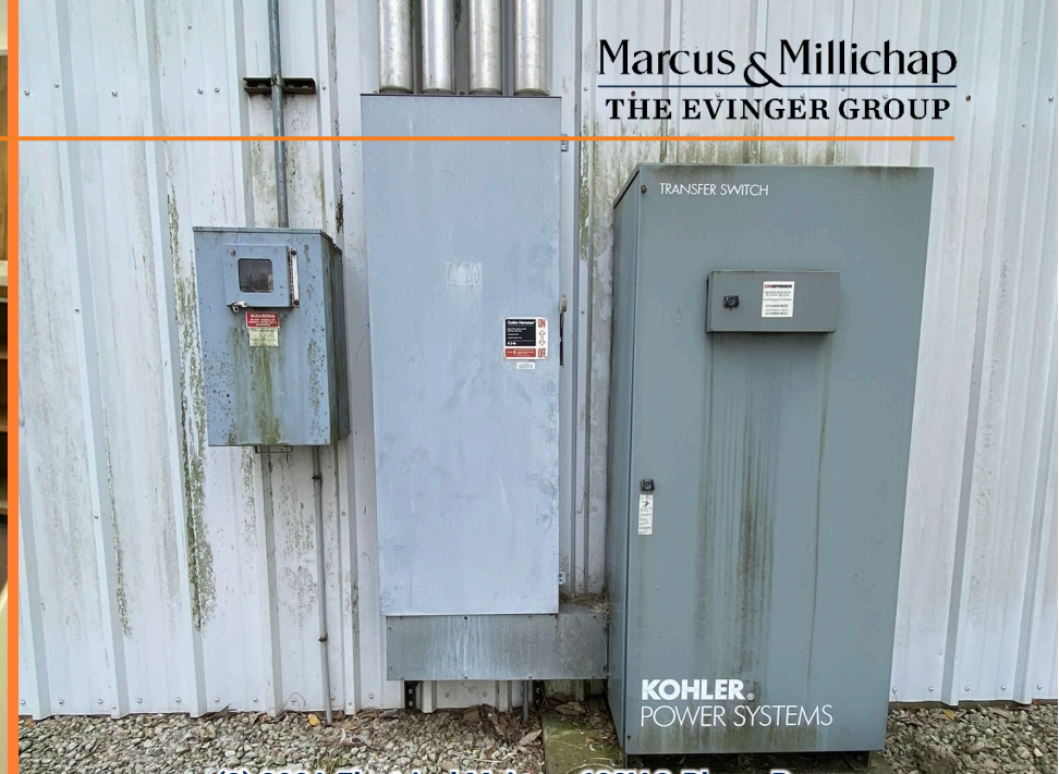
(2) 800A Electrical Mains - 600V 3-Phase Power
