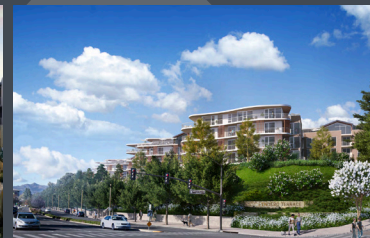
Lindero Terrace - 693 apartments
