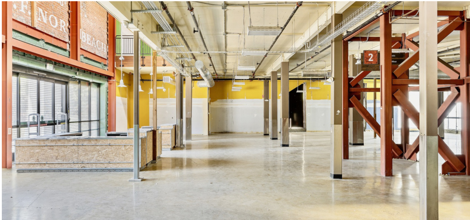
Annex Building (2598 Taylor)
