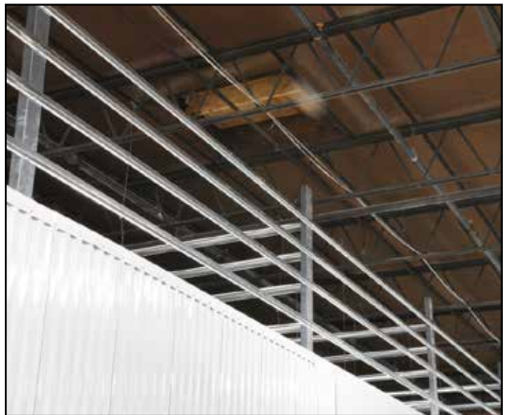
8a. Burglar bars can also be supplied above partition panel to divide every unit.
