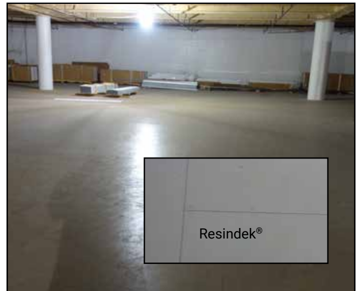
13b. Resindek® paneling installed over "B" deck.
