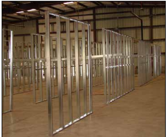
11a. Multi-floor galvanized studs are installed 30" on center.
