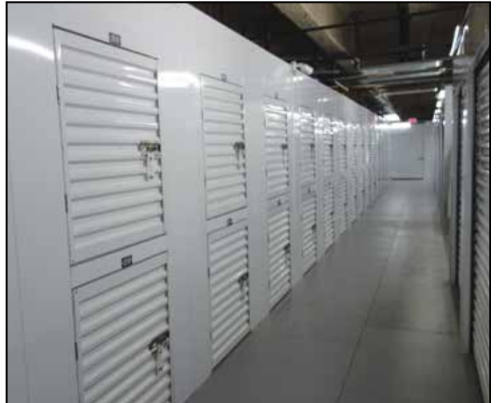
3a. 5' W X 5' D X 4' H locker, double stacked with 3'0" X 3'4" colored swing door.
