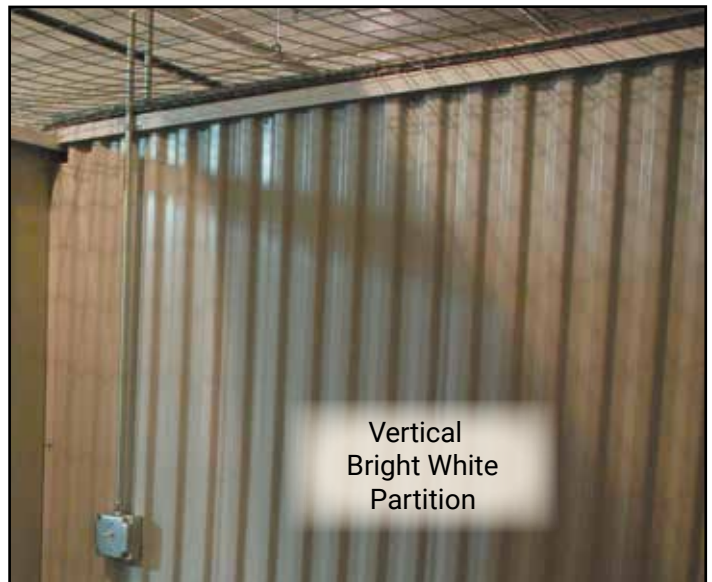
6b. Vertical bright white rigid-rib panel is an alternative to the galvalume partition panel. This is widely used in apartment conversions.
