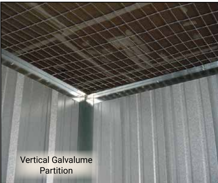
6a. Interior units consist of vertical galvalume partition panel with galvanized interior angles .
