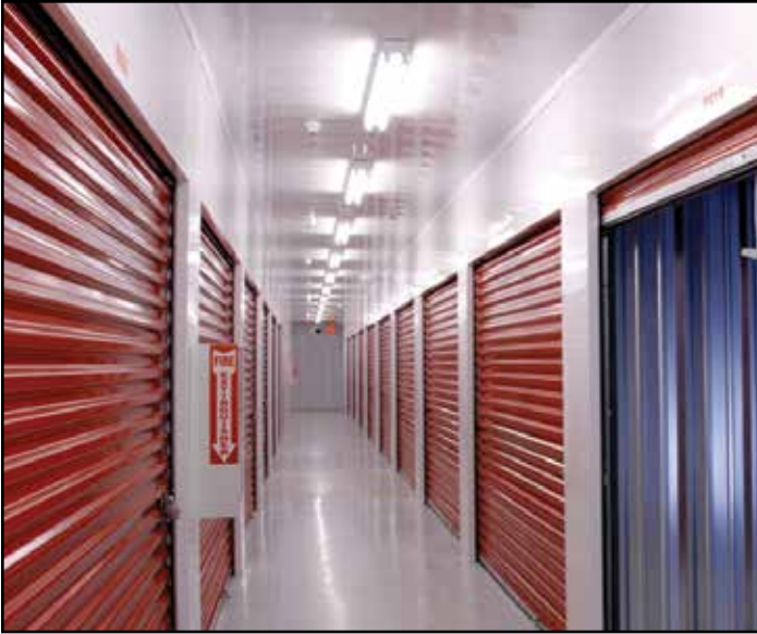
5b. A bright white flush ceiling covers all interior duct work and completely encloses the corridor, resulting in a clean, finished look. Lights can be installed directly to the ceiling panel.
