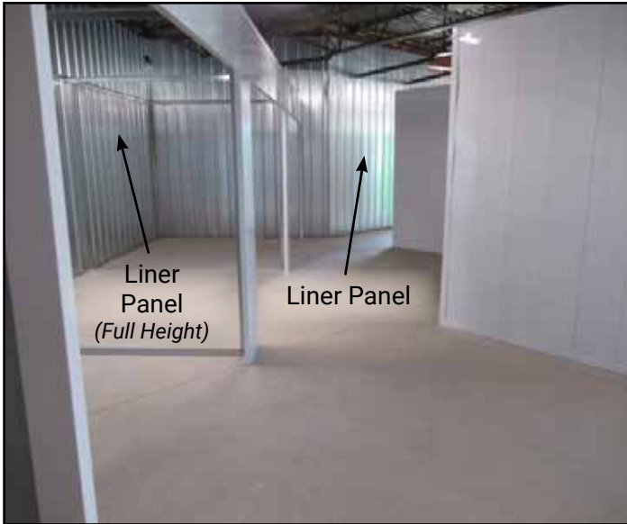
9a. 29 gauge vertical galvalume liner panel can be installed on perimeter walls. They can be installed to unit height or full perimeter wall height.
