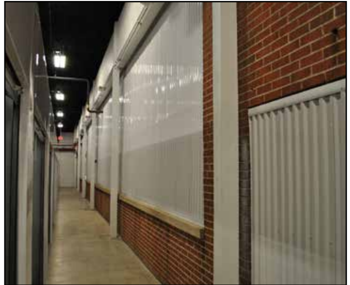
9b. 29 gauge vertical bright white rigid rib panel can be installed on perimeter walls located next to corridors. A bright white semi-flush panel is an alternative to the rigid rib panel. They both can be installed to unit height, full perimeter wall height or at custom heights shown above.
