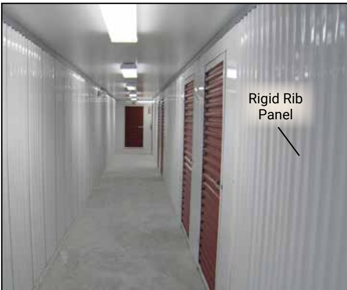
2a. Trachte standard partition corridor uses a bright white rigid-rib hallway panel for all blank walls. (An optional center girt can be ordered to stiffen the wall.)
