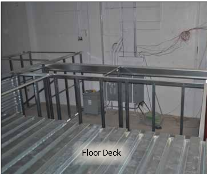
13b. Galvanized "B" floor deck which is smooth to accept Resindek® floor paneling system.
