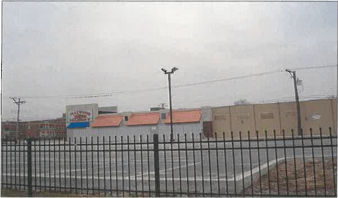
WESTERN BUILDING ELEVATION AND PARKING LOT
