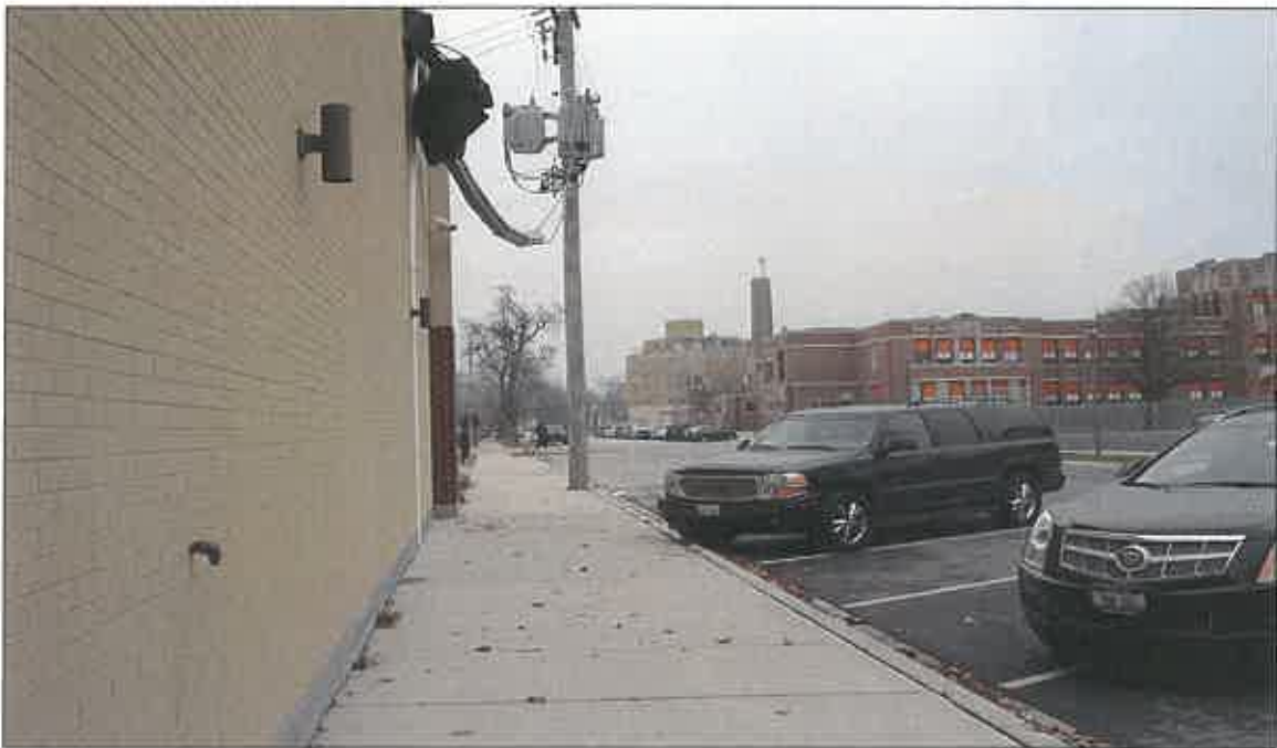
EASTERN BUILDING ELEVATION
