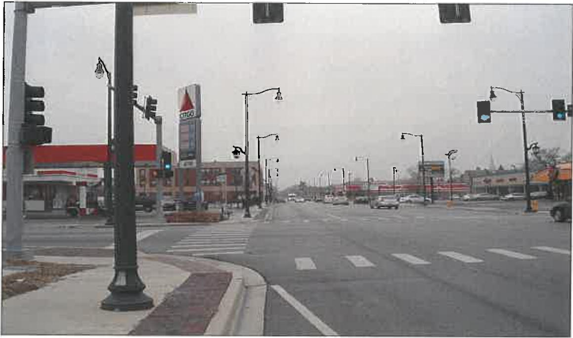
VIEW SOUTH IN 5TH STREET - SUBJECT AT LEFT
