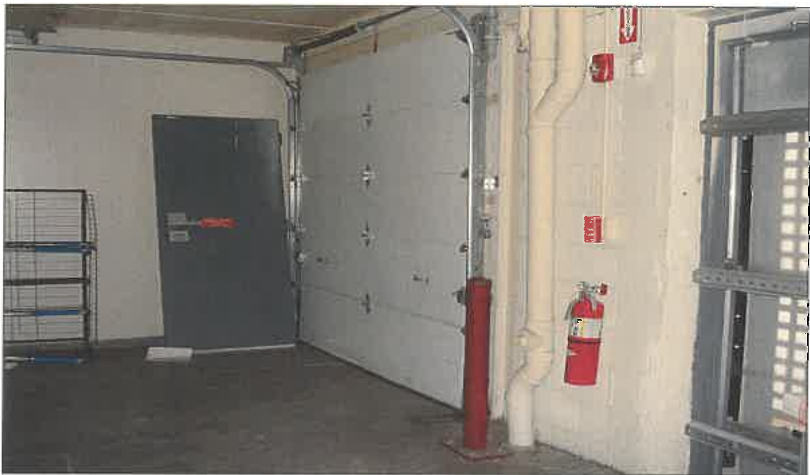
DRIVE-IN DOOR – LOADING AREA
