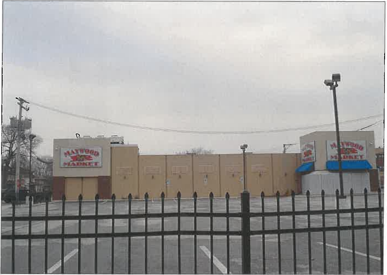
NORTHERN BUILDING ELEVATION AND PARKING LOT
