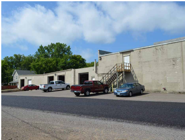
East Side of Building w/ OH Doors
