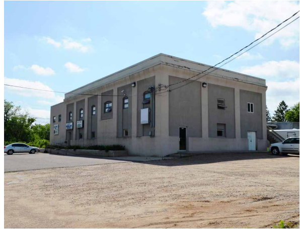
NW Corner of Building
