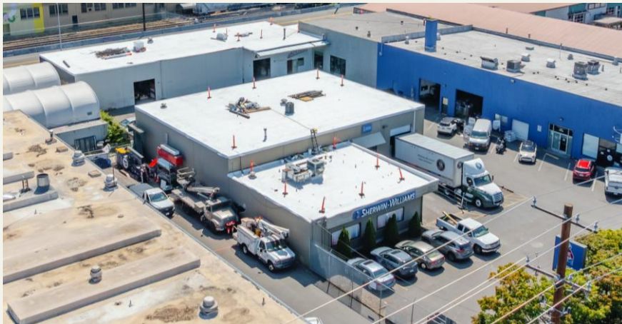
*Roof work actively in progress at time of photo
