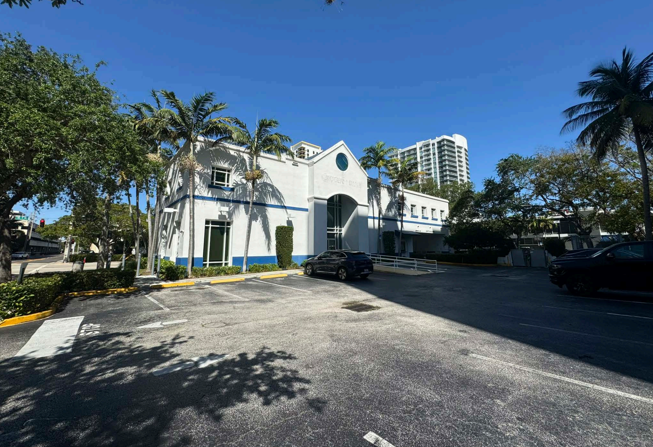
200 NE 3RD AVENUE | EXTERIOR PHOTO
