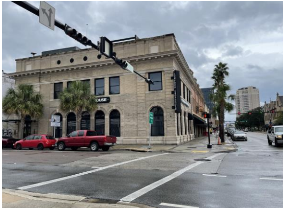
Front view of the subject building. Photo was taken November 22, 2023
