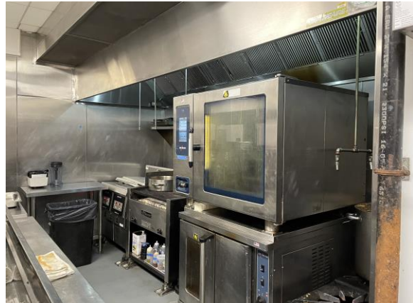
Kitchen Area (2 nd Floor) Photo was taken November 22, 2023
