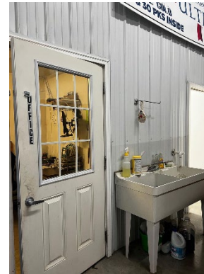
1 st Fl. Office Door
