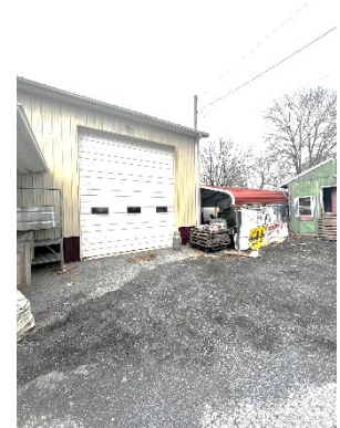
Warehouse Bay Door
