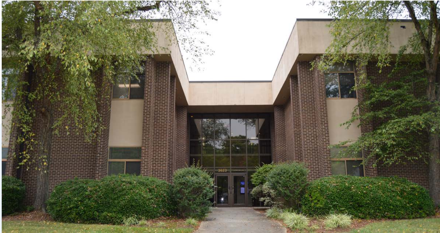
Front Entrance of 3623 Latrobe Drive.
