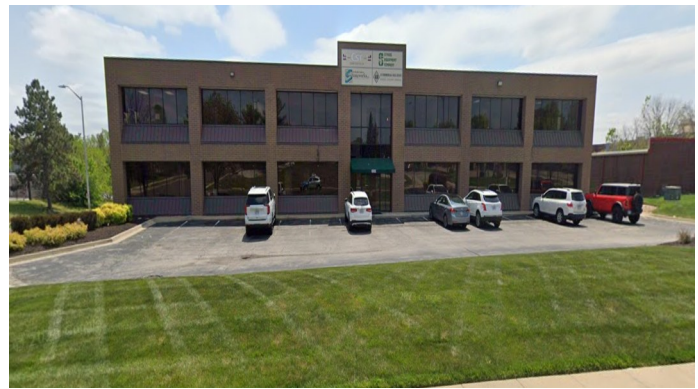
North View of Building
