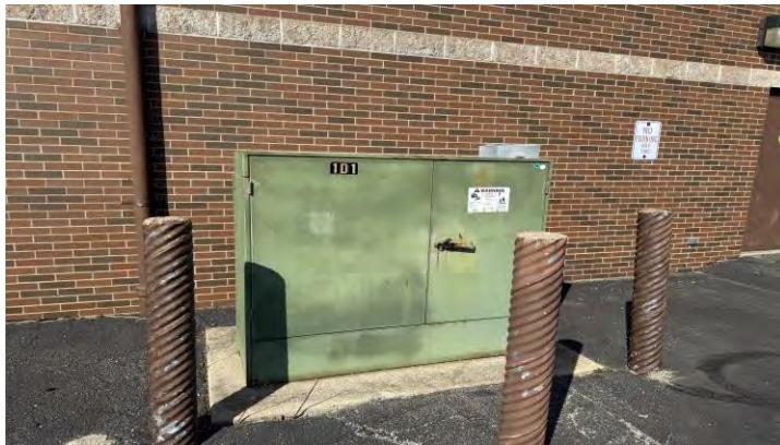
**Photograph 15: Pad-mounted transformer observed on the southern portion of the Property**
