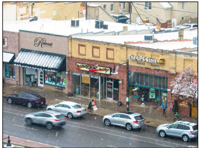
Snow covered building featuring central AC
