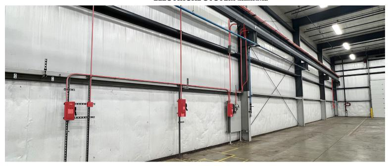
Facility includes (18) 3-phase distribution points throughout the building. Perfect for running heavy machinery and manufacturing equipment. All 480V which can be stepped down to 120/208V.
