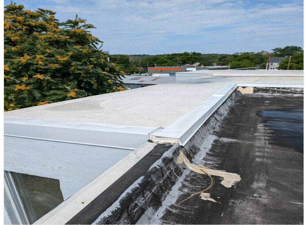
photo of roof over suites 103 and 104 - July 2024
