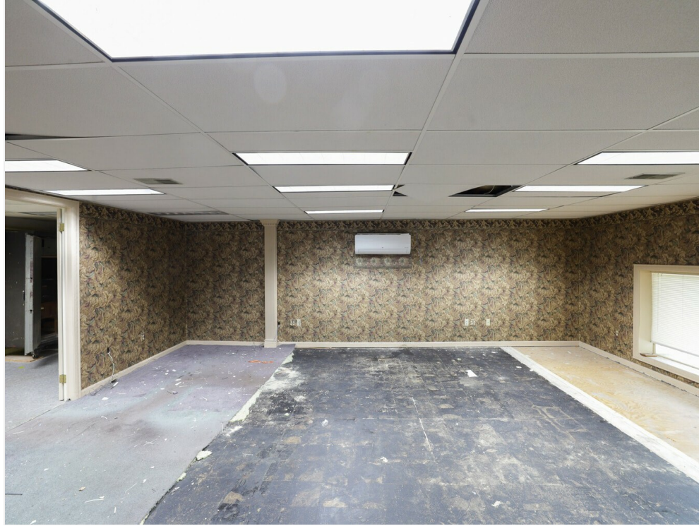
second floor office space - unit 201
