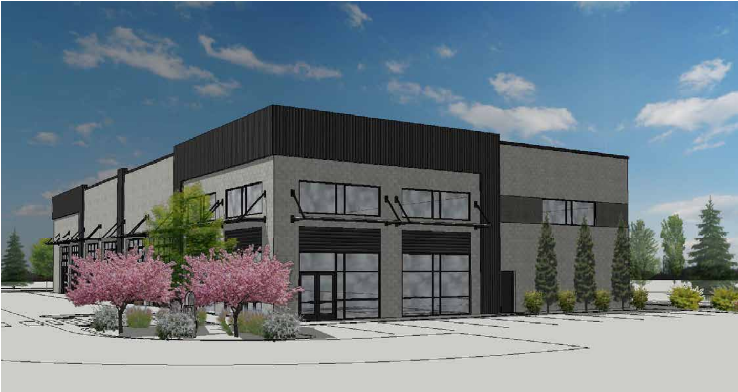
Aerial View Looking Northwest
