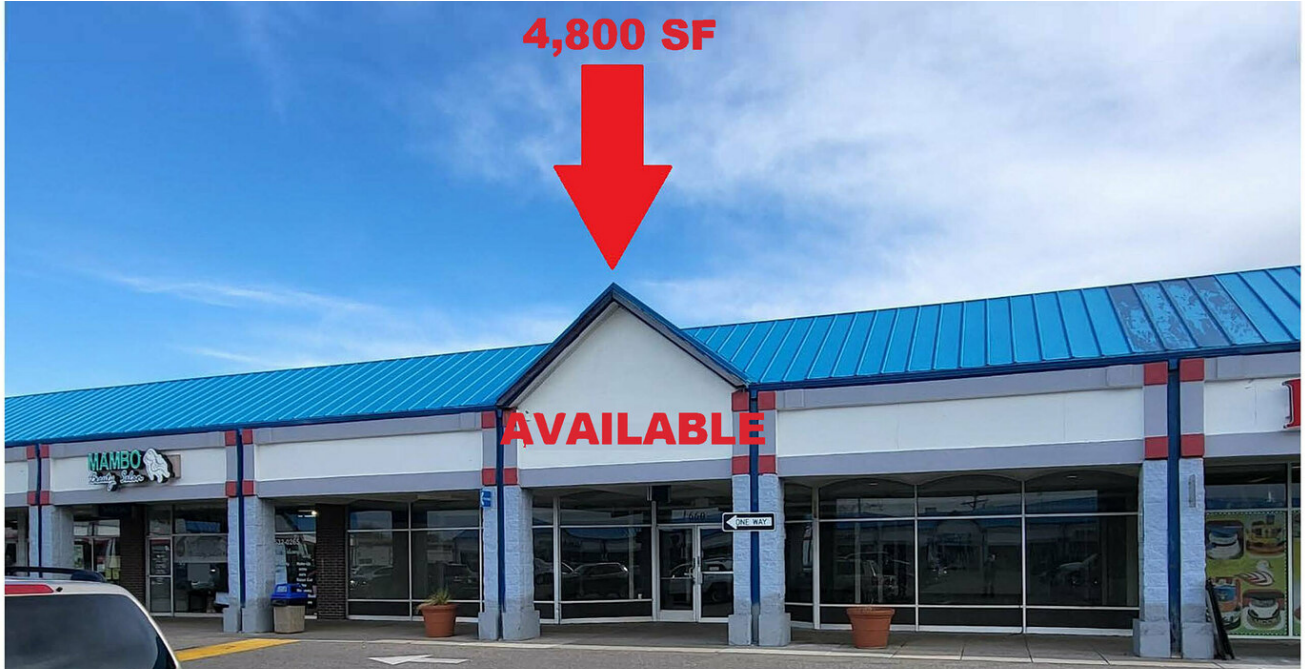
660 Peoria exterior view looking south
