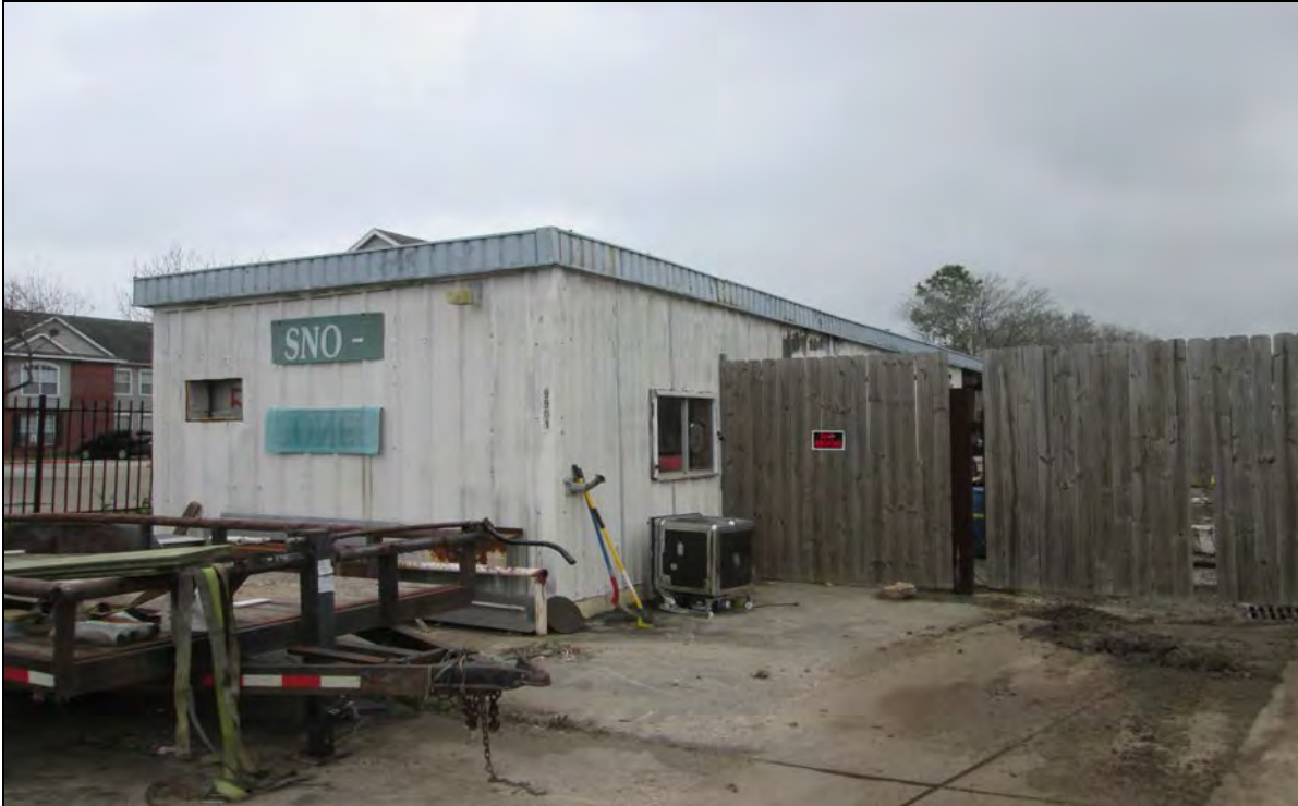
Standing on the southwest portion of the subject, looking at a view of the metal storage building.
