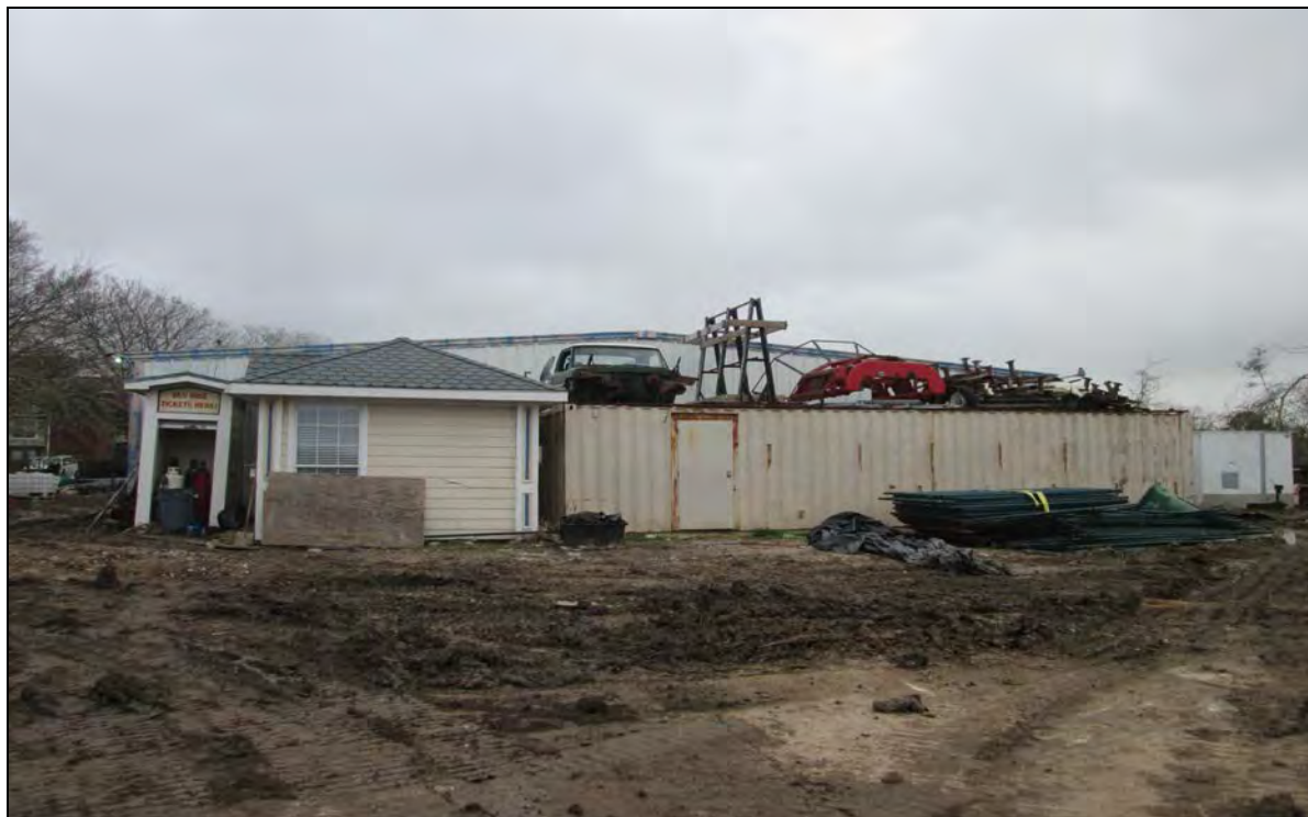
Standing on the subject property, looking north at a view of the breakroom building and metal shop.
