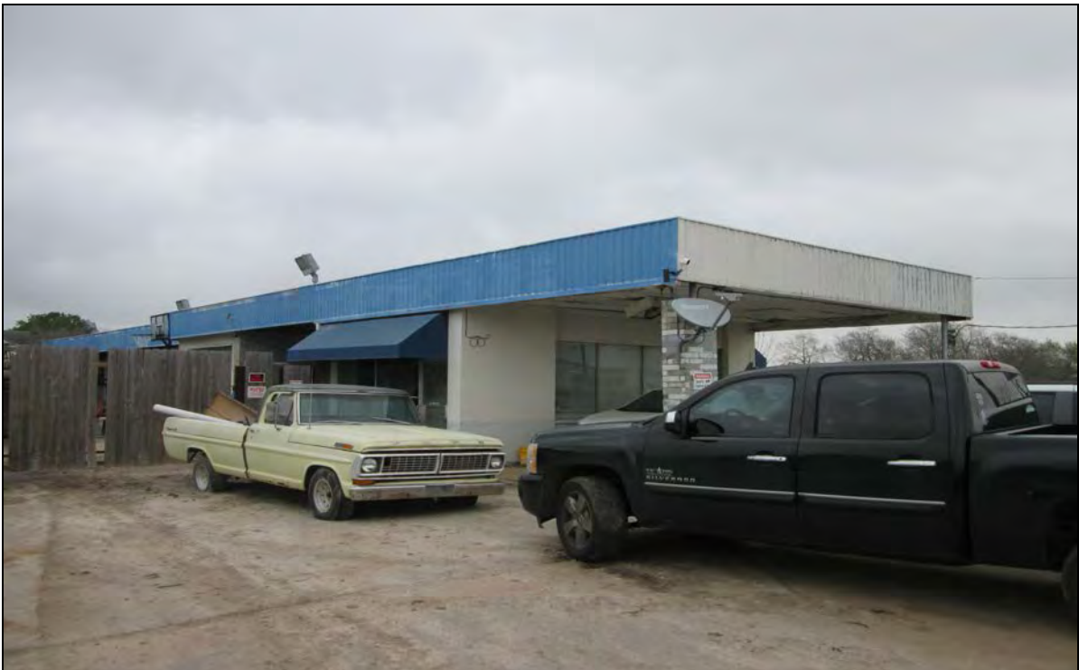
Standing on the southwest portion of the subject, looking at a view of the office building.
