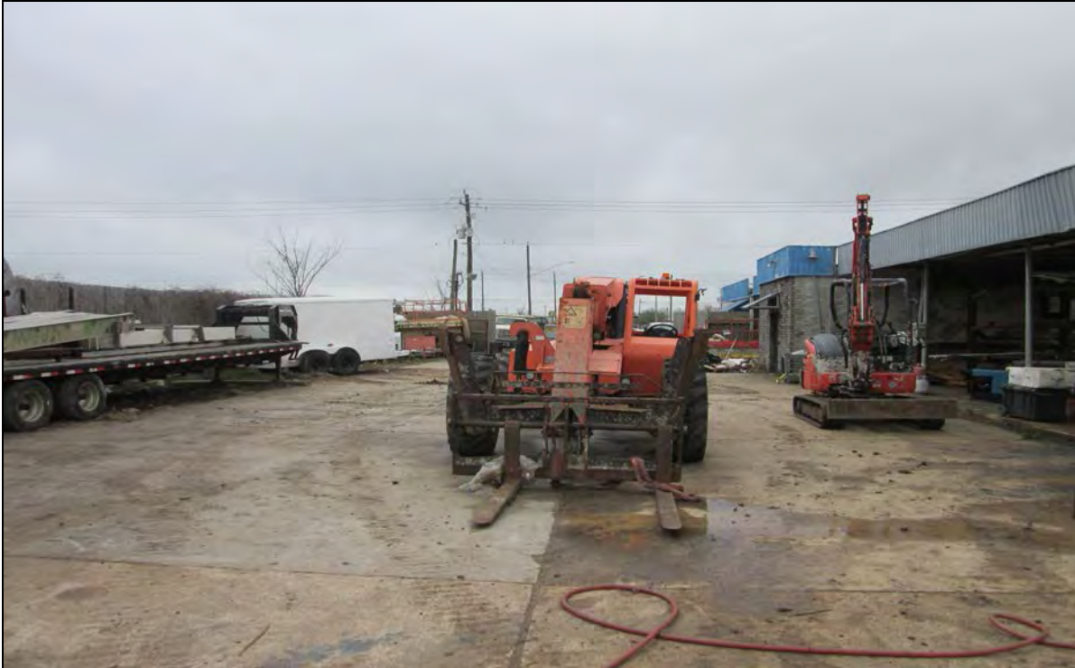
Standing on the subject property, looking at a view of the subject.
