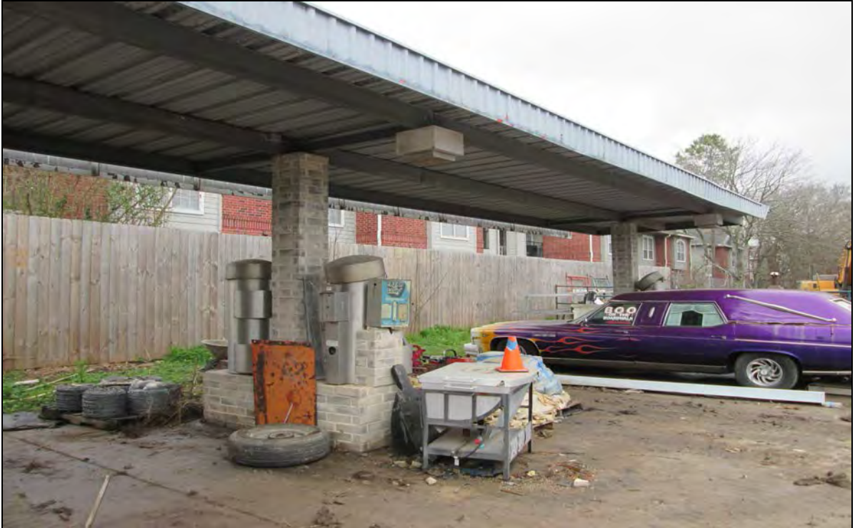
Standing on the subject property, looking at a view of the metal storage building canopy.
