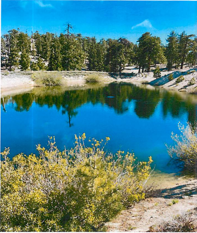
4 Million Gallon Snow Making Reservoir
