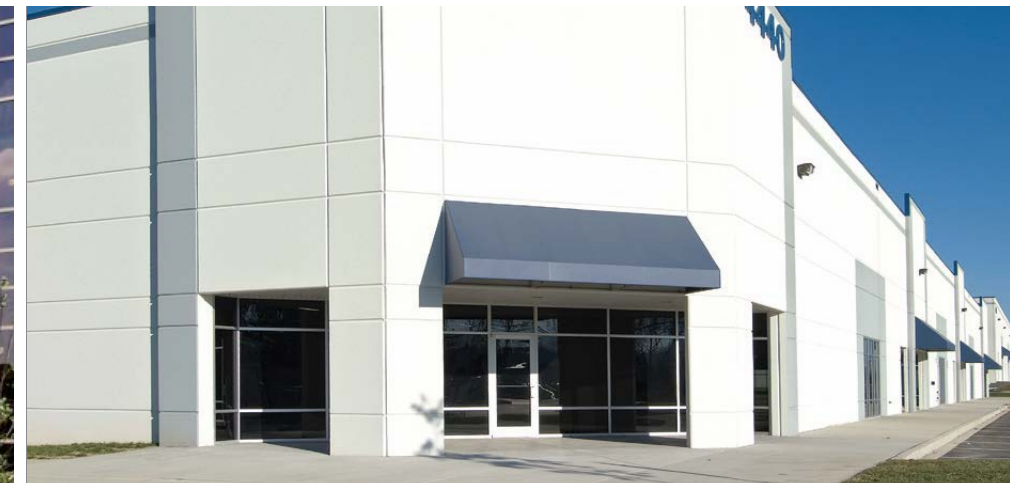
Federal Emergency Management Agency Wedgewood South – High Bay Warehouse
