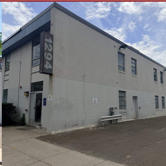
Rear Elevation & On-Site Parking Lot
