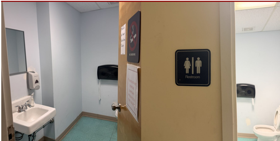
Restroom — Interior with Sink
