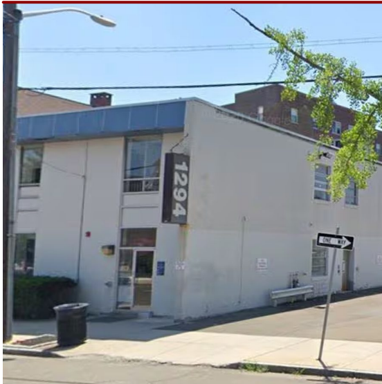
Street-Facing Facade — 1294 Chapel Street
