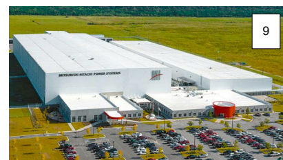
9 MITSUBISHI-HITACHI POWER SYSTEMS
