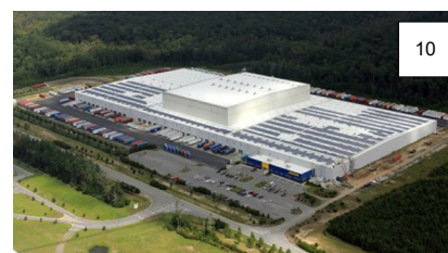
10 IKEA DISTRIBUTION CENTER
