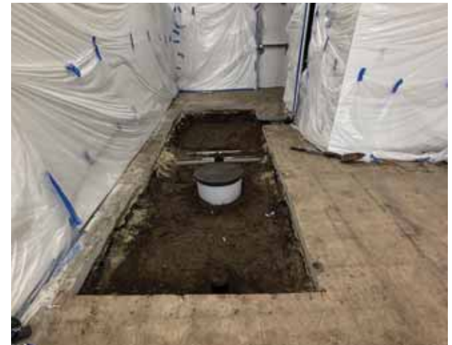
1122 Interior - Inground 40-Gallon Grease Interceptor
