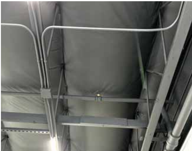
1122 Interior - Open Beam Ceiling
