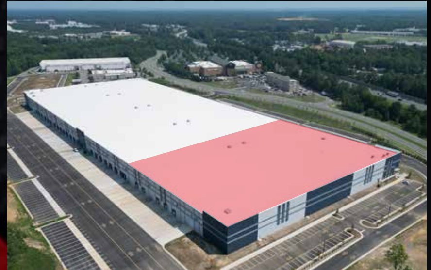
As-built Office Suite
