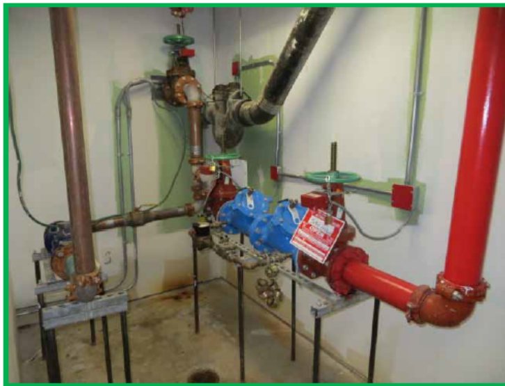
SPRINKLER CONTROL VALVES
