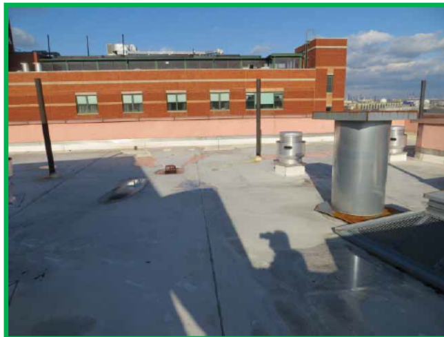
VIEW OF THE ROOF
