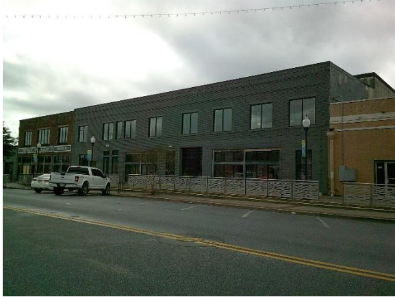
Front View – Subject Property
