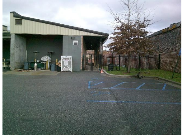
Rear View – Subject Property
