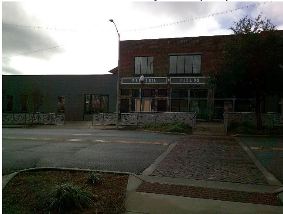
Front View - Subject Property
