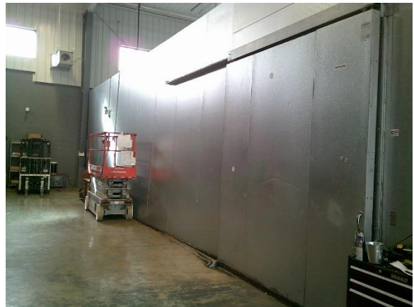
Interior View – Cooler
