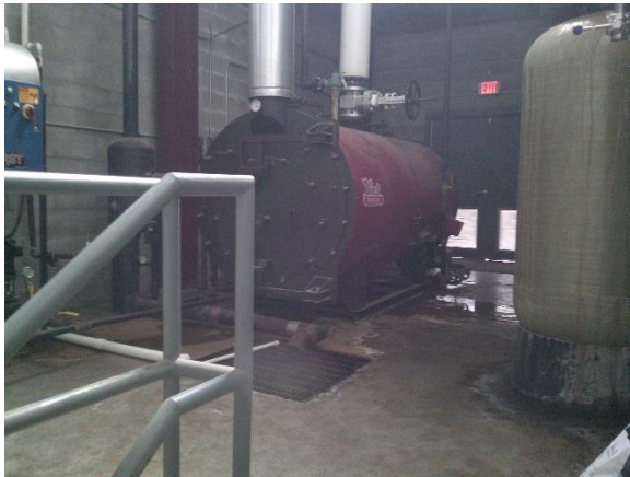
Production Area – Subject Property
