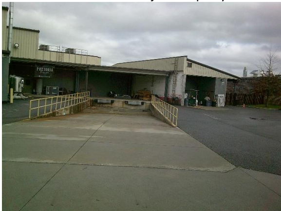
Rear View – Subject Property
