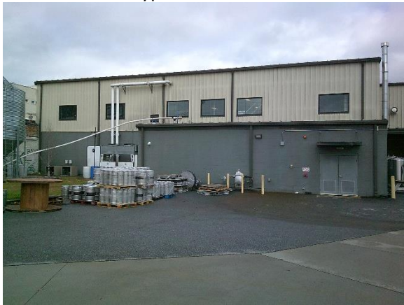
Rear View – Subject Property
