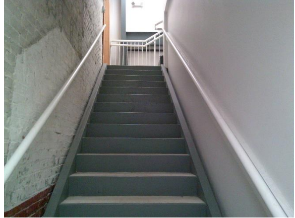
2 nd Floor Access Stairs
