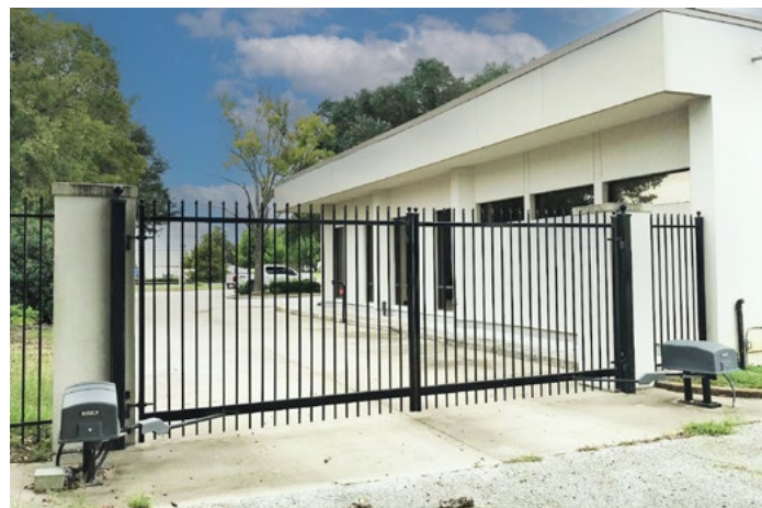
SECURED PARKING GATE
