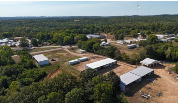
Old Hwy 71 Storage
