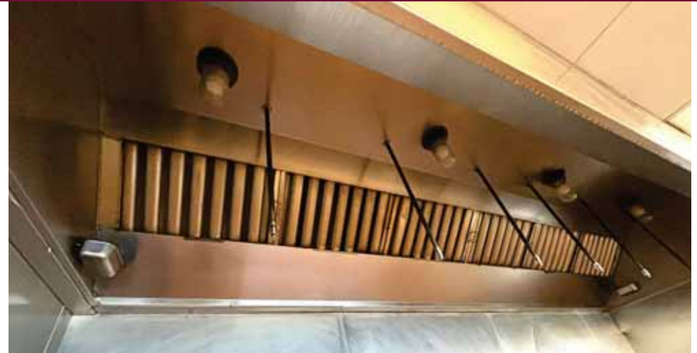
1795-#60 - Type 1 Stainless Steel Exhaust Hood
