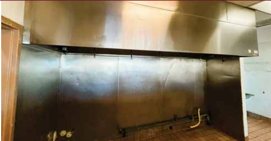
1795-#60 - Type 1 Stainless Steel Exhaust Hood
