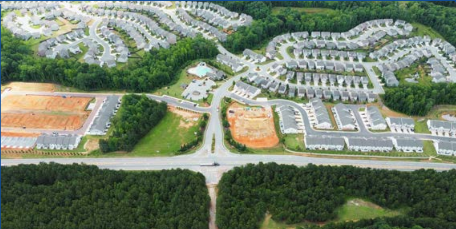
AUBURN STATION DEVELOPMENT ACCESS
