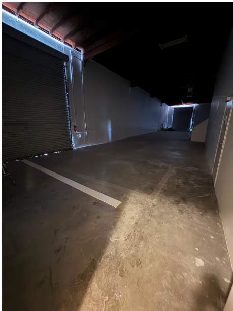
WAREHOUSE — GROUND LEVEL DOOR
