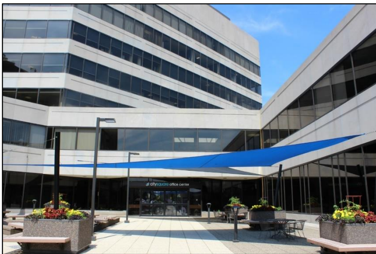
Main Building Entrance (Floor 2)
