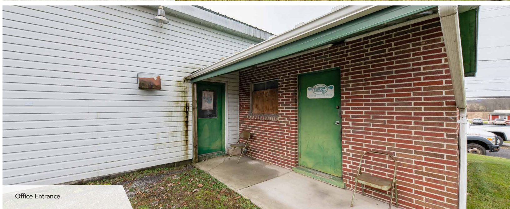
Front and Side of Building.
