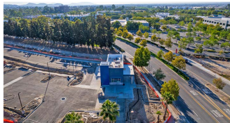
ACTUAL SITE - UNDER CONSTRUCTION
