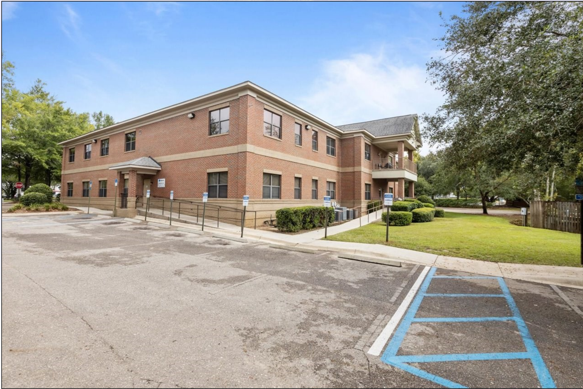
Exterior View (North Side)
