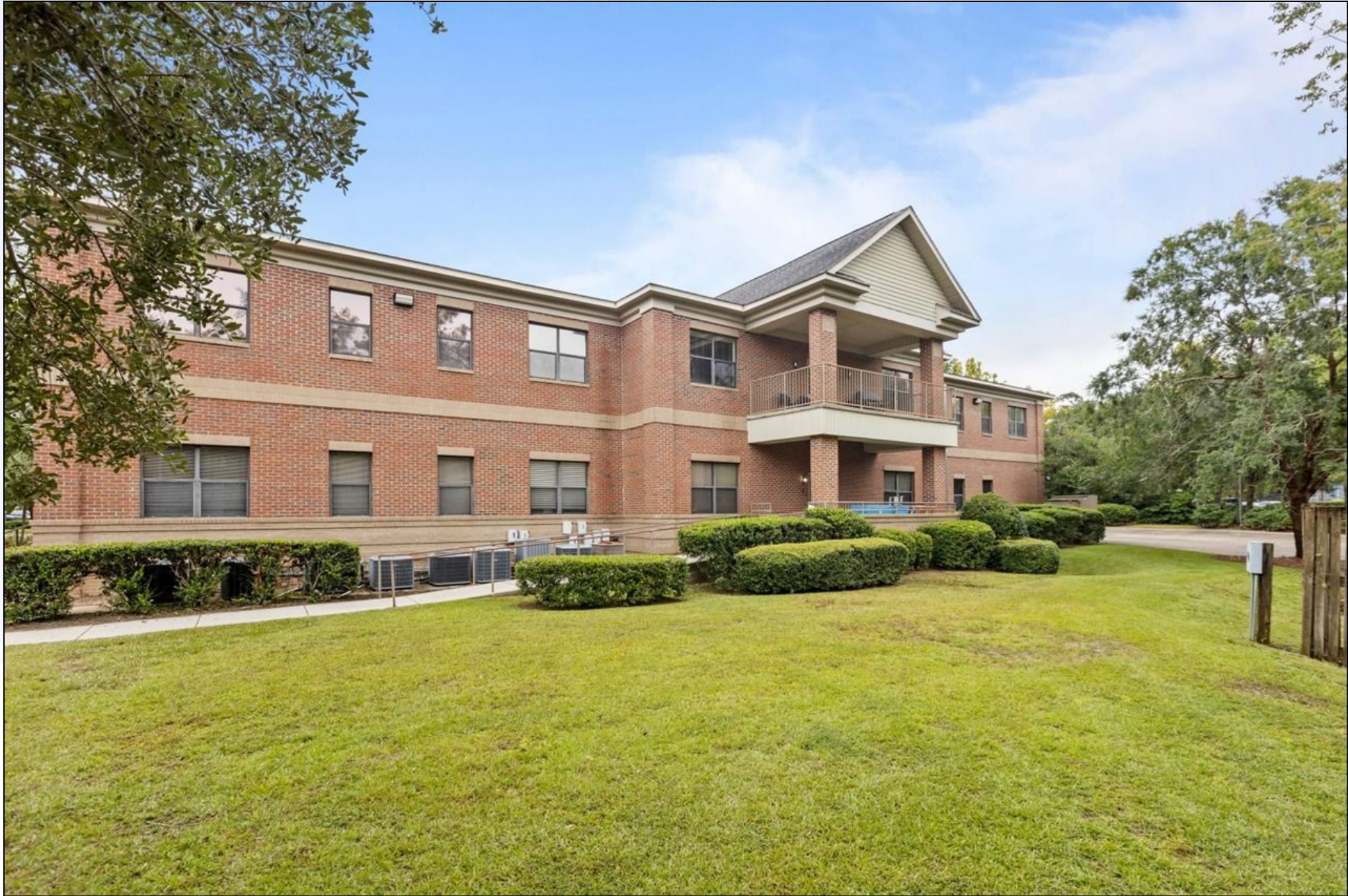
Exterior View Rear (Showing Covered Porches)
