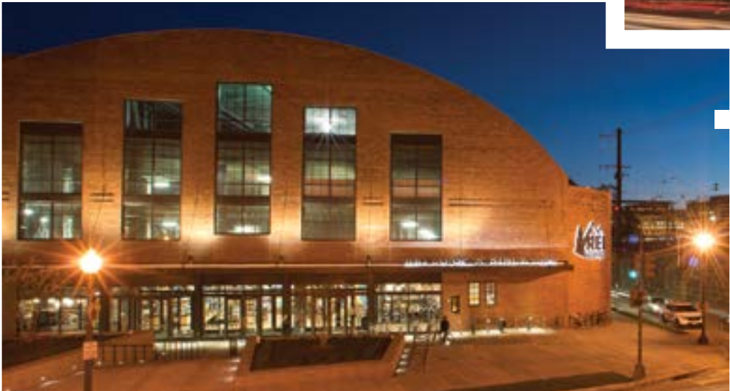
ULINE ARENA, DOUGLAS DEVELOPMENT, DC
