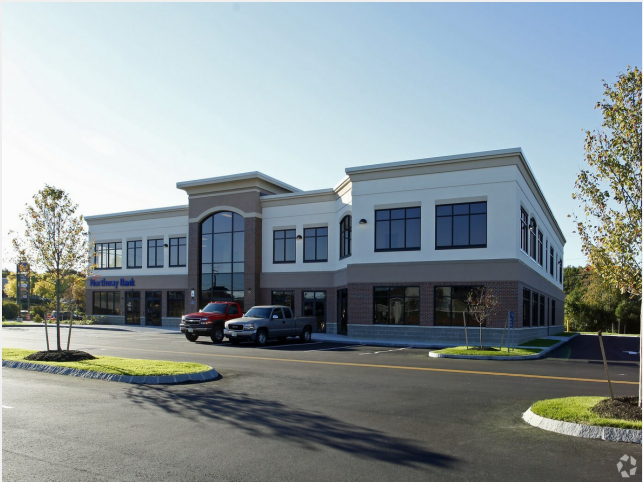
5 units in building 1
