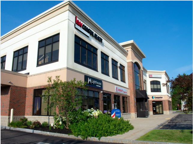
Bank space with drive through ATM
