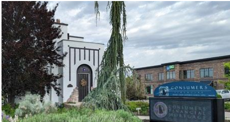
Art Deco Entrance & Monument Sign
